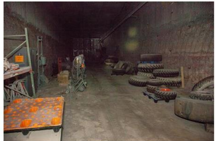
Combustible Loading in the Mine
