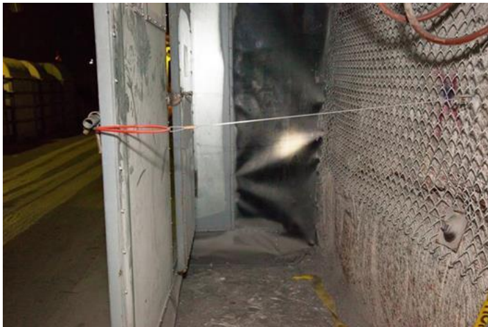
Air Lock Doors Wired Open
